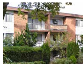
1929 West 3rd Avenue Vancouver
